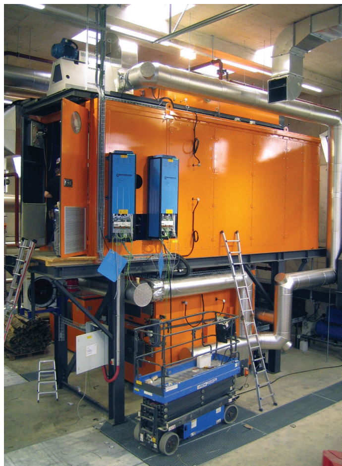
The heat-to-power cogeneration system with hot-air turbine in the central energy station of the district heating network of Dürdingen. Photo: Schmid AG
