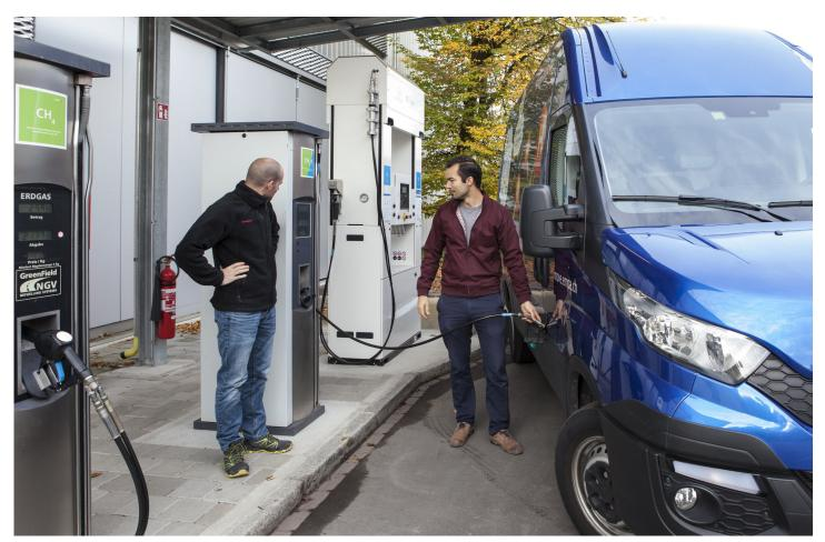
The three fuel dispensers of the "move" project at Empa provide different fuels: methane (front), a methane-hydrogen mixture (middle) and hydrogen (rear). Photo: Empa
