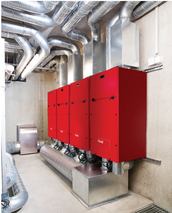
Comfort ventilation ensures good air quality in air-conditioned and wind-tight buildings. Photo: Hoval
