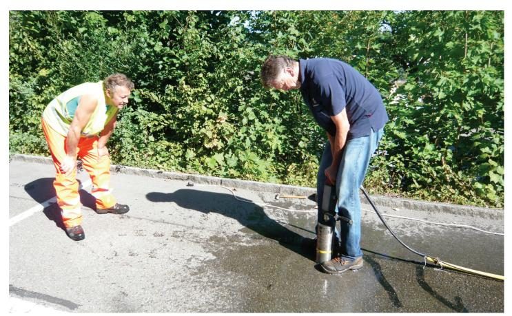
The Internet of Things includes, for example, sensors that record the occupancy of parking spaces and report the information to the parking guidance system. In the photo, drill work for the installation of sensors in a pilot project in Lenzburg. The battery-powered sensors require only one borehole, no further cabling is necessary. Photo: Swisscom, André Portner
