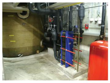
The heat exchanger (blue) absorbs the heat from the solar circuit and supplies it to the groundwater, which is stored in the groundwater tank (brown). Photo: B. Vogel
