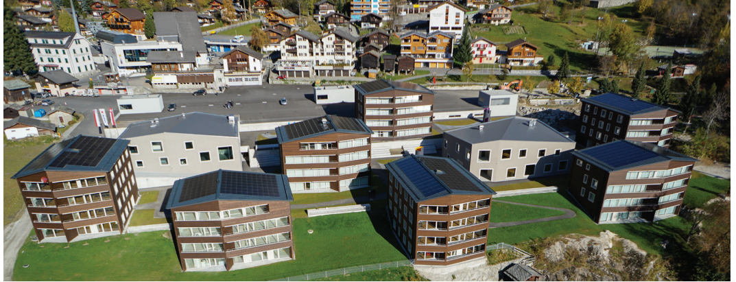
The roofs are oriented to the west and east. The solar yield falls in the mornings and in the afternoons and when energy use peaks in the village (during the day the holiday guests are usually not home). Photo: Lauber IWISA AG
