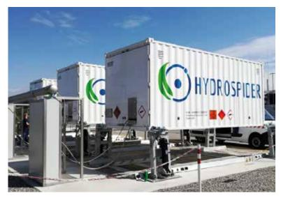
A 2MW electrolyser plant at the run-of-river power plant "Gösgen" will go into operation in 2020 to produce "green hydrogen" for fuel cell trucks. The picture shows tank containers, where the hydrogen produced is temporarily stored and which are used to supply the filling stations in Switzerland with hydrogen (Source: Hydrospider).
