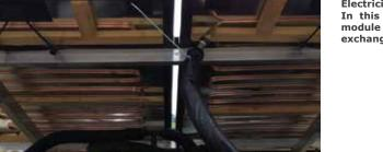
Electricity and heat for a heat pump: In this example a conventional PV module was retrofitted with a heat exchanger (source: ZHAW).
