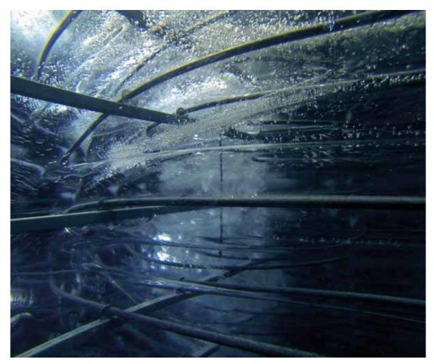
Underground ice storage system with a heat sink capacity of 30,000 kWh. Ice storage systems are latent heat storage systems with water as the storage medium, where the latent heat is used as storage during the phase transition from ice to water and vice versa. In the temperature range above 0 °C, they can also serve as sensitive heat stores (source: SCHNEPF Planungsgruppe Energietechnik, Nagold, Germany).
