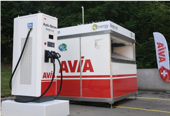
This hydrogen-powered pilot charging station was used 30 times to charge an electric vehicle in St. Gallen during the project period from March to August 2022. The vehicles took an average of 27 kWh of energy, with an average charging time of 34 minutes. For this purpose, green hydrogen was used, which had previously been produced using renewable electricity from hydropower by means of electrolysis. Photo: H2 Energy
