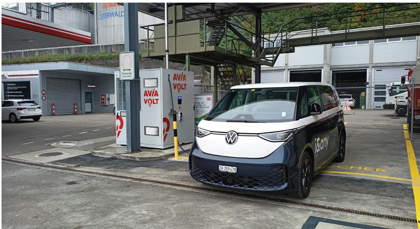
Under the name “kvyreen 80,” a hydrogen-powered charging station for electric vehicles with a charging capacity of 80 kW was put into operation in St. Gallen in October 2023. Photo: H2 Energy
