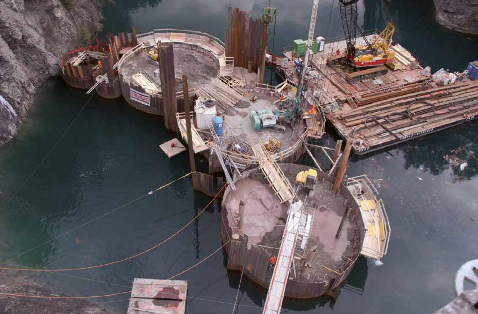
*Construction of the sediment diversion shaft at the Solis reservoir on the Albula in the canton of Grisons.*
