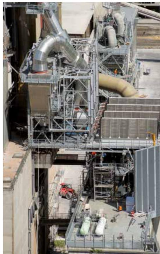
**Waste heat from a cement factory can be used for producing electricity with the aid of an ORC (Organic Rankine Cycle) system.**
