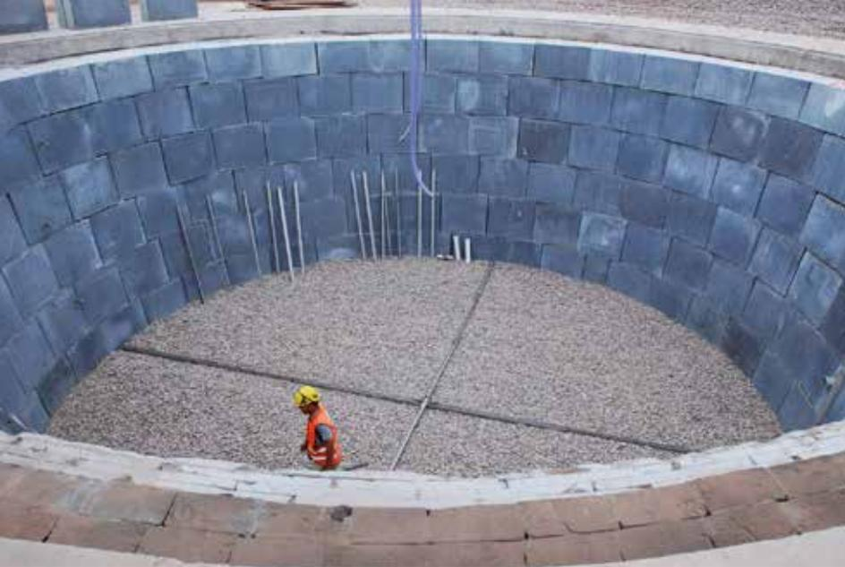
**Basalt thermal storage system for surplus solar heat.**
