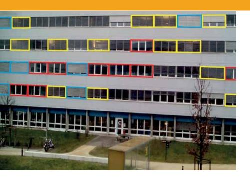
West facade of an office building with manually operated blinds on a cloudy day: use of blinds is random and only a few are in the appropriate position (shown in red). The lights are on in some of the offices with the blinds partially drawn (shown in yellow).
