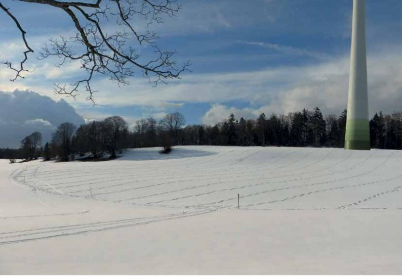
Transects in the snow in a radius of 100 metres around a wind turbine at the Peuchapatte plant, which were used for carrying out searches for collision victims
